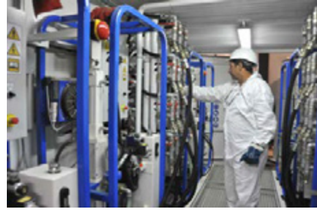
Fig. 4 automatic grouting plant
