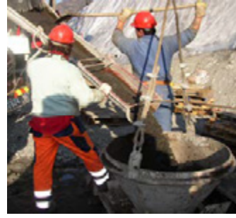
Fig. 2 ZVI poured into the excavation
