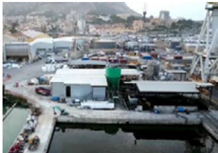
Fig. 7 Aerial view of the job site
